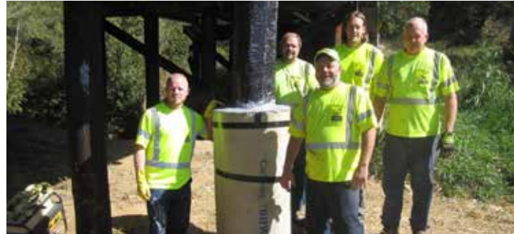
Repaired pile on KY 32 over Blaine Creek in Lawrence County, Ky. Photo courtesy of University of Kentucky.
