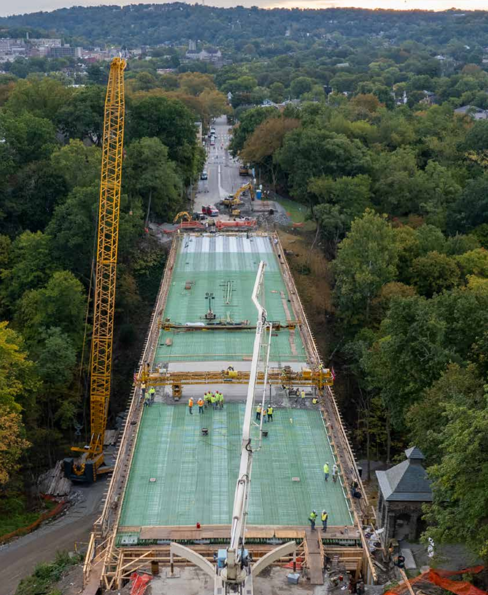
Fern Hollow Bridge construction. Photo courtesy of HDR, Inc.
