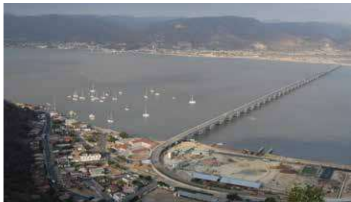
Bahia Bridge in Ecuador. Photo courtesy of Earthquake Protection Systems (EPS).
